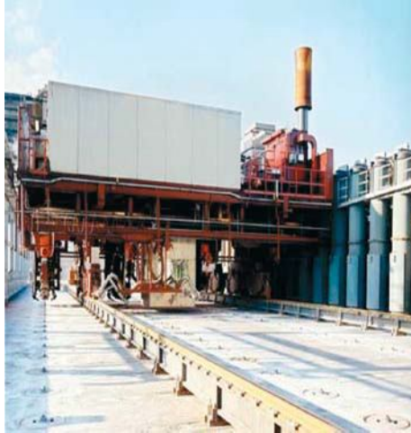
Coke charging car
